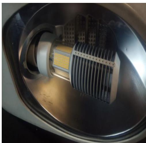
(a) 150W HPSV light fixture with an LED lamp
