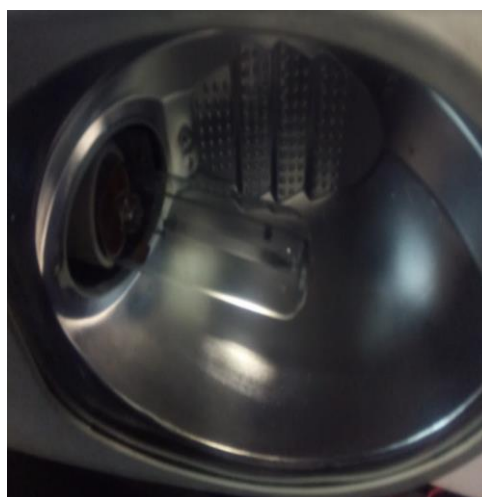
(b) 150W HPSV light fixture with a 150W HPSV lamp inside
